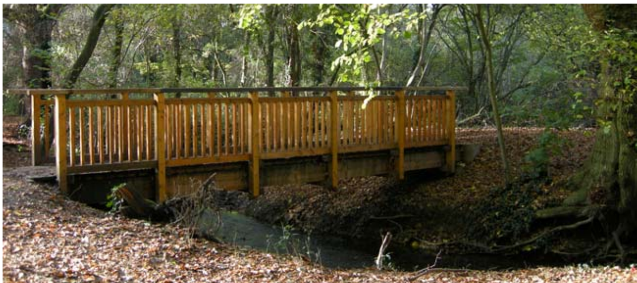
Completed new footbridge over Toddbrook in Netteswell Plantation
